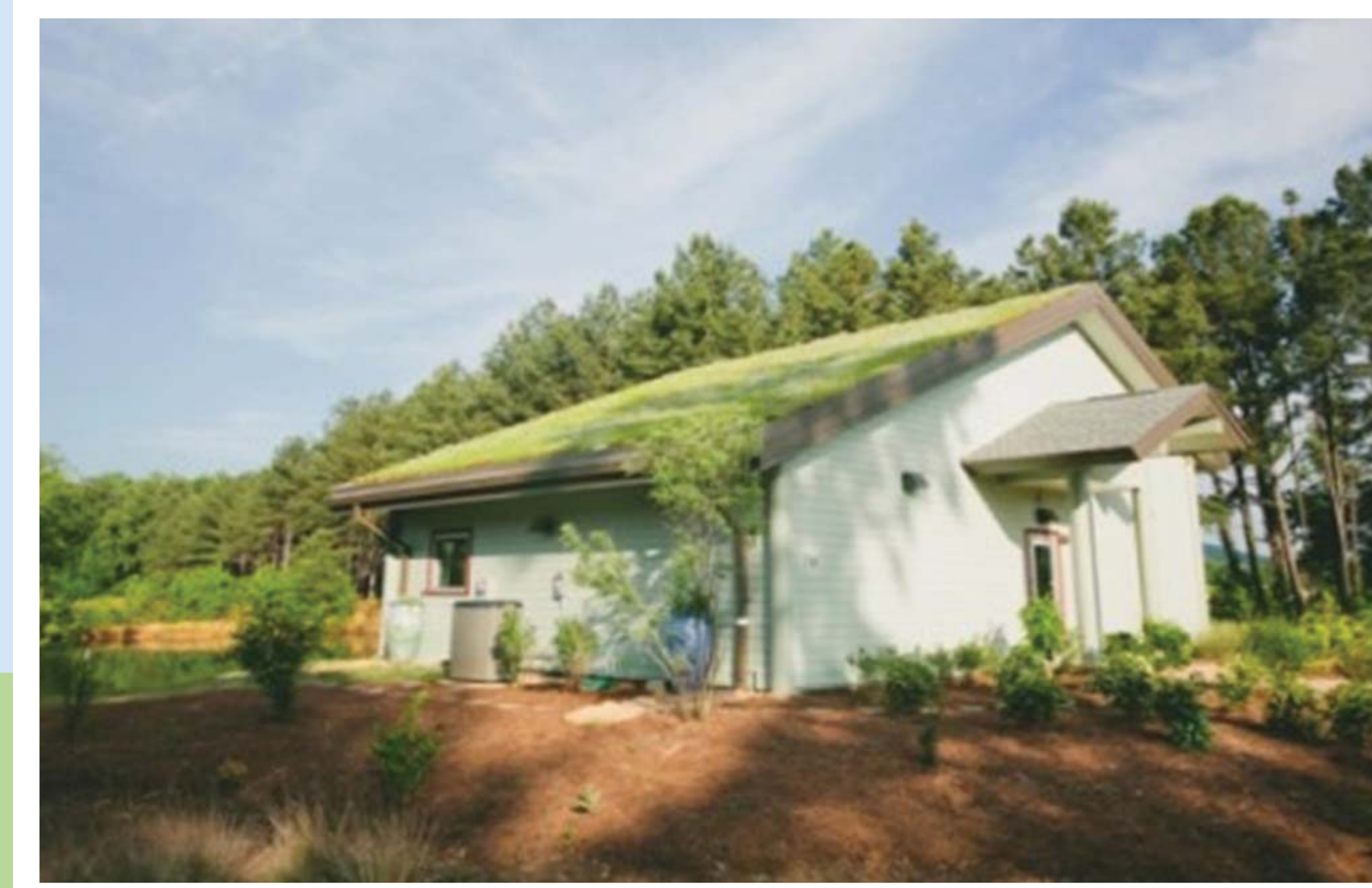
(right) Green Roof, Hays Nature Preserve, Huntsville, AL (Courtesy – Jerry Cargile, 4Site, Inc.)
