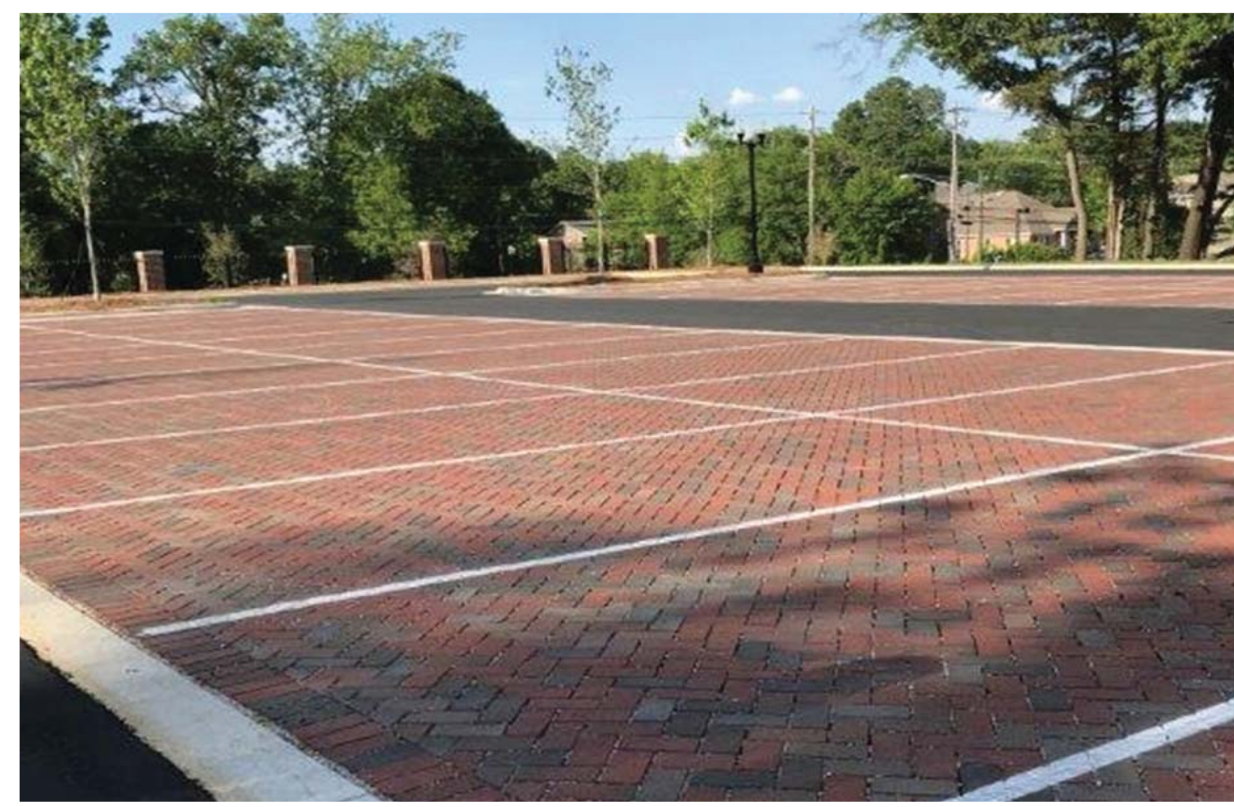
Permeable Pavers and Bioretention, East Glenn Public Parking, Auburn, AL
